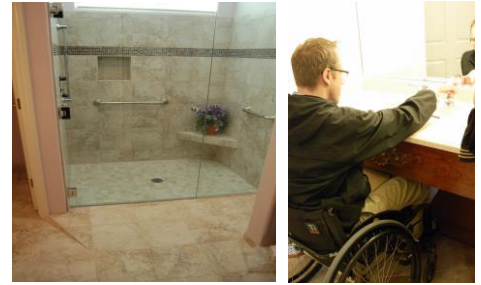
An adapted roll in shower with grab bars and a handheld shower head (left), and a sink with space to wheel under (right). 11-12
