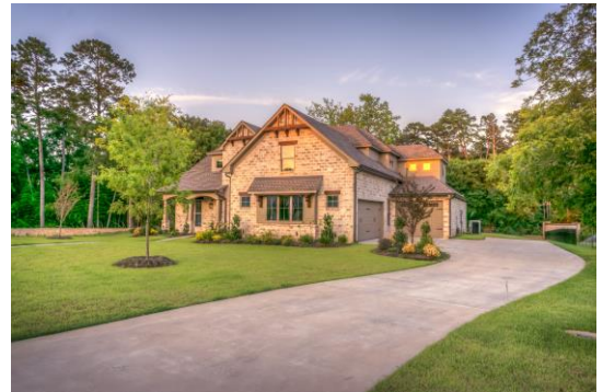
A house built with universal design includes no steps/stairs from the start. 7
